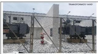
Without power transformer, the pumping station cannot just use the high voltage from electric wires directly; Meanwhile, the low voltage electric power cannot transfer to us directly by the power transformation system. Therefore, the transformers are used to control the flow of power as per the requirement of input and output devices of the pumping station
