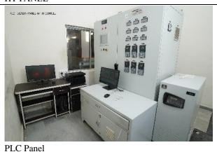
**Programmable Logic Controllers (PLCs)** are small industrial computers with modular components designed to automate customized control processes. PLCs are often used in factories and industrial plants to control motors, pumps, lights, fans, circuit breakers and other machinery. Integrated **PLC Panel** can monitor any process and provide data wherever and however you need it.
