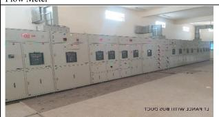
Low Tension Panel is an electrical distribution board that receives power from generator or transformer and distributes the same to various electronic devices and distribution boards
