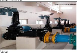
Valves are used for regulating the flow and pressure within a piping system and for improving safety through relieving pressure or vacuum in a piping system
