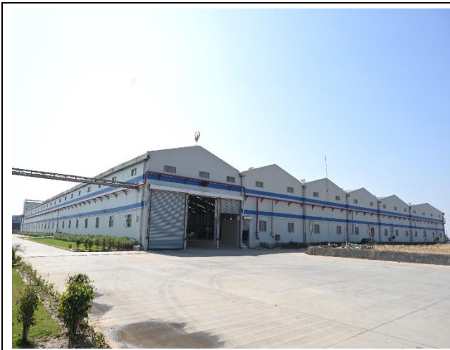
MANUFACTURING PREMISE ENTRY
