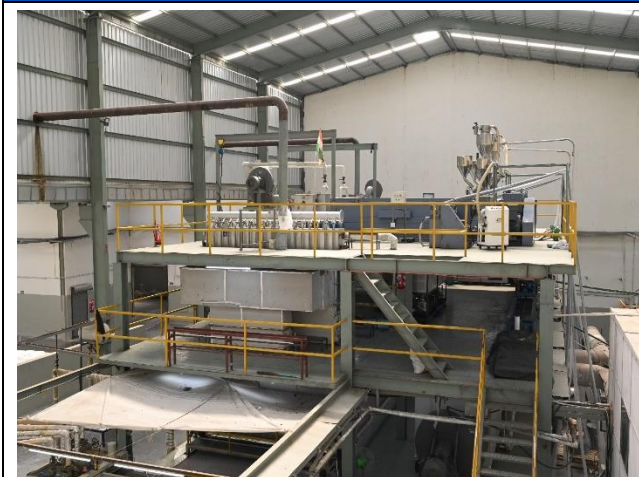
MIXING AND PROCESSING AREA
