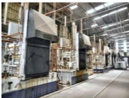
Heat treatment line
